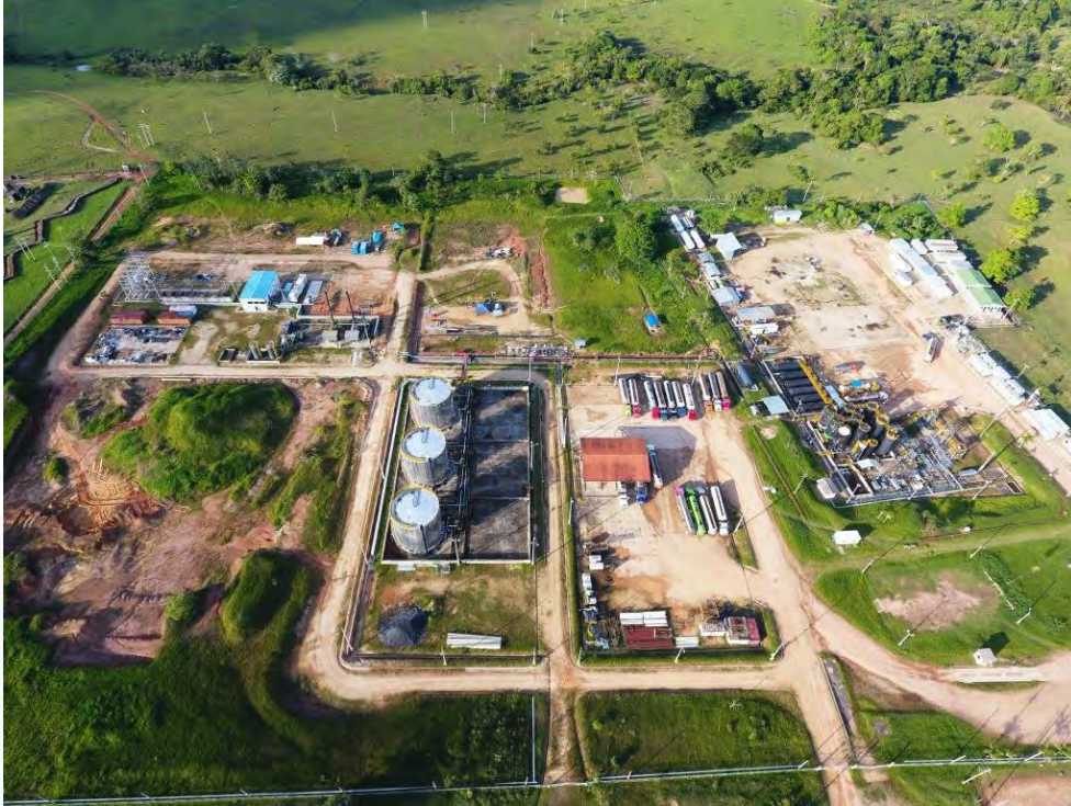
Figure 9 - Capella Central Processing Facility and Pad A
